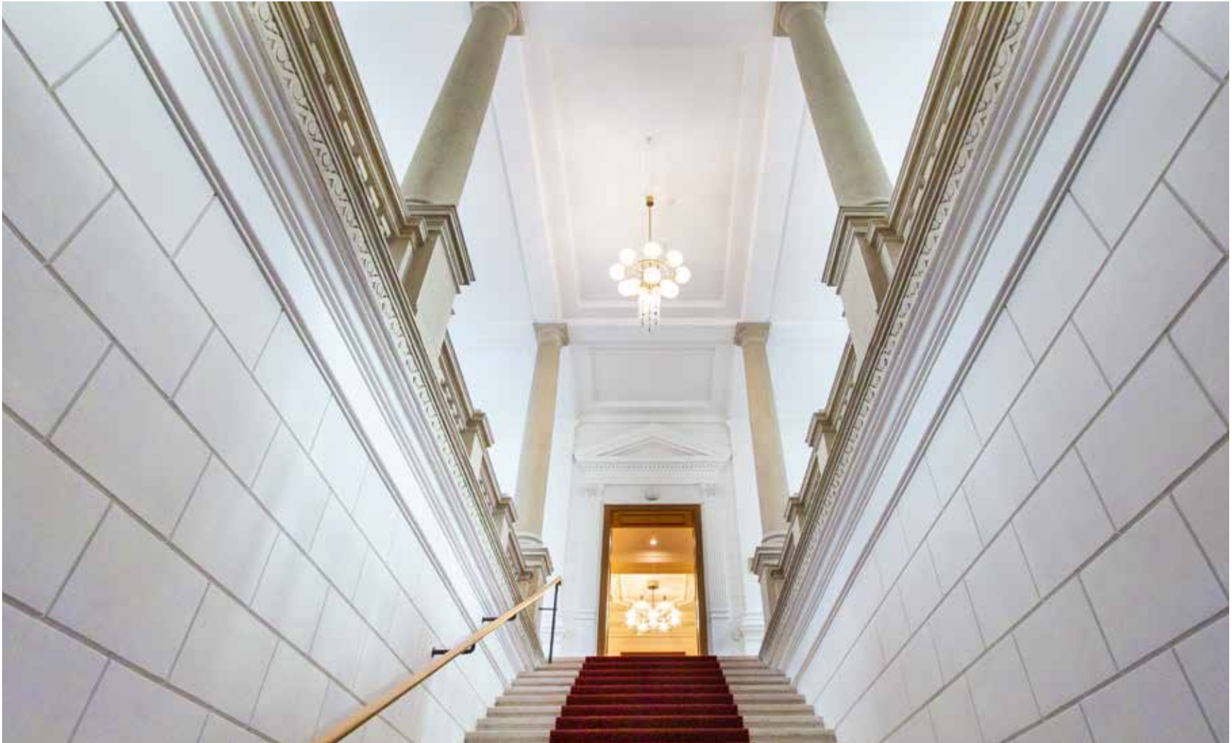
Missing handrails were added to the existing staircases
