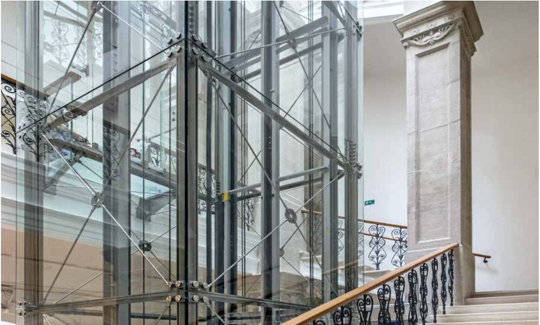
The construction of the new lift was a sensitive matter; the equipment and technology did not disrupt the existing architectural appearance
