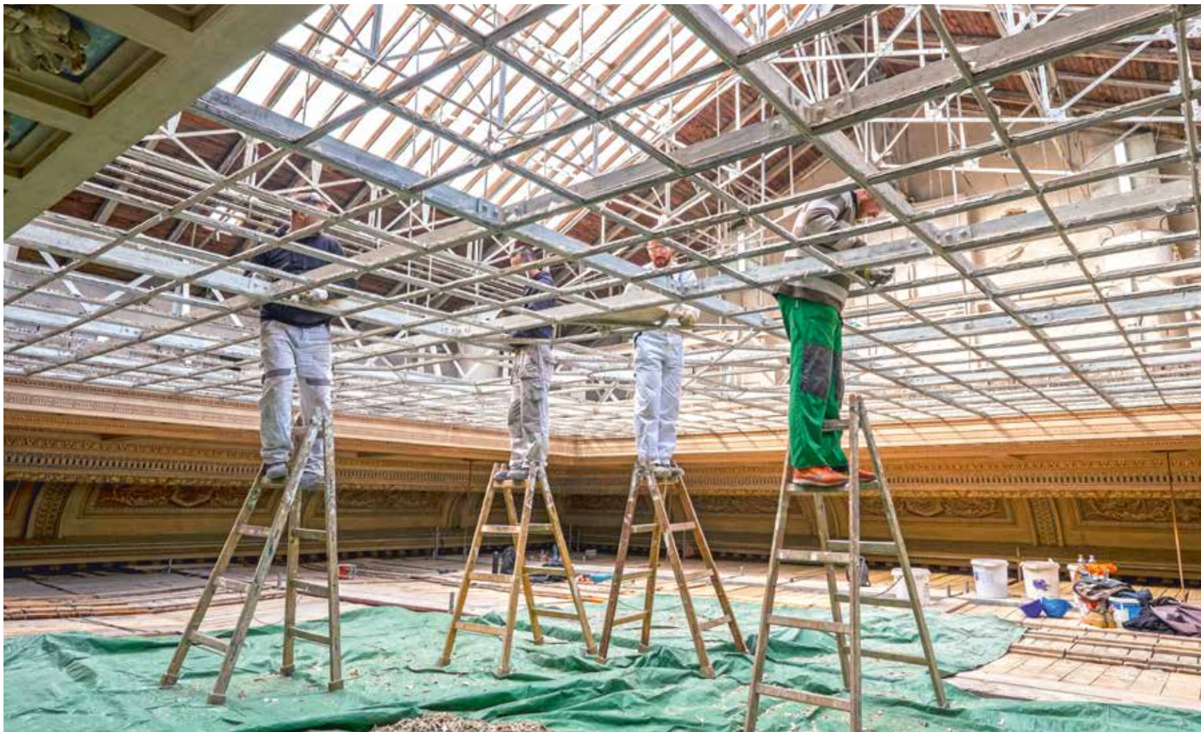
Renovation of the roof light's metal structure
