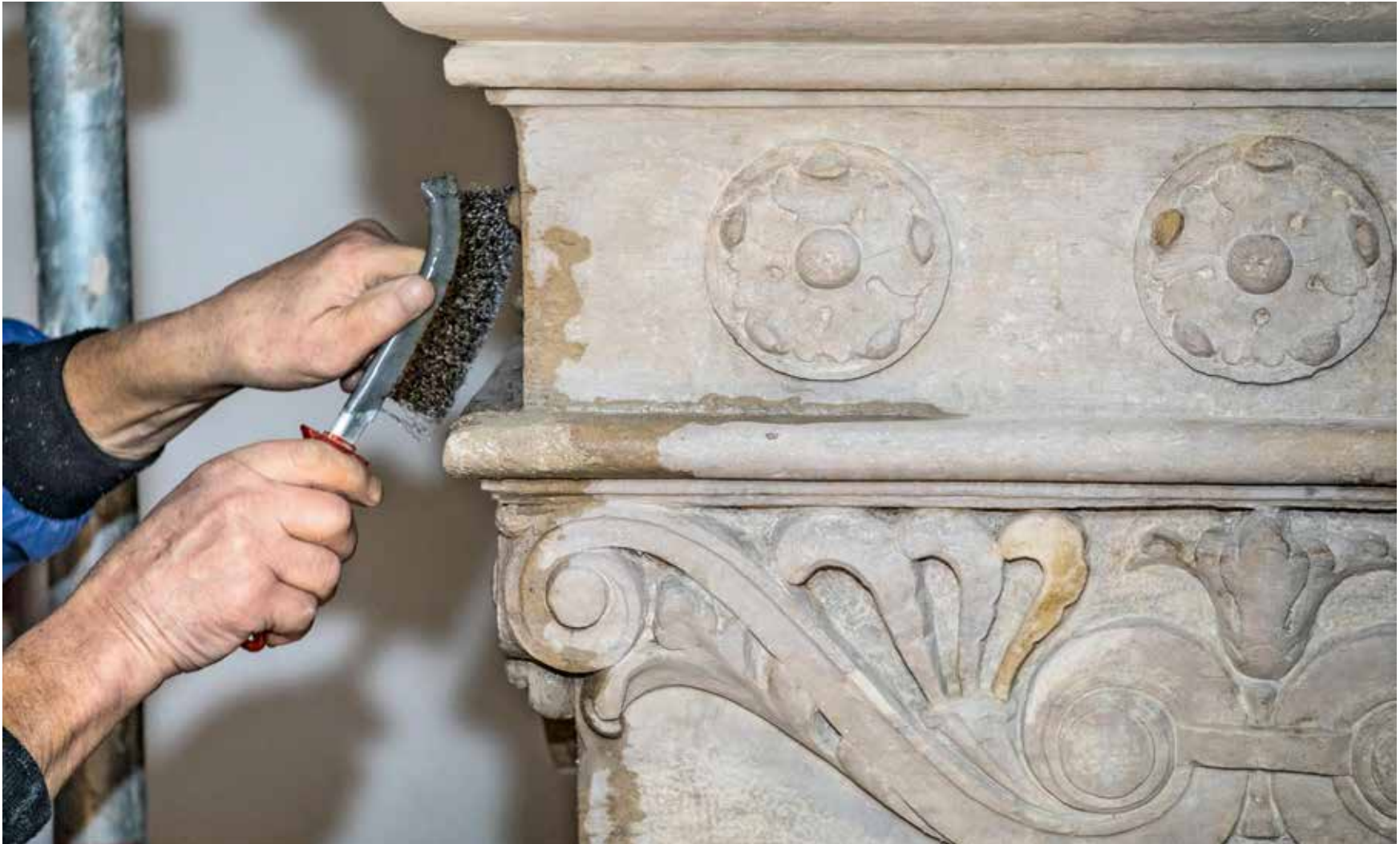
Renovation and restoration works in the staircase area
