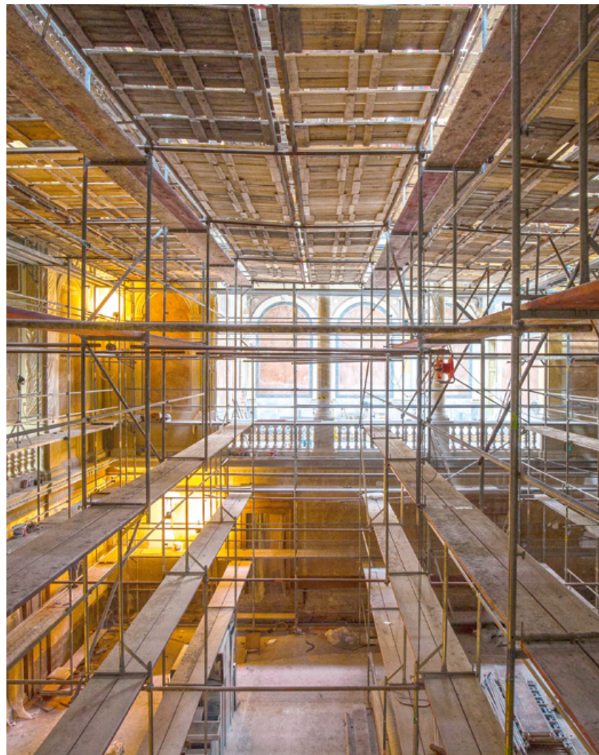
The Assembly Hall in the course of reconstruction works
