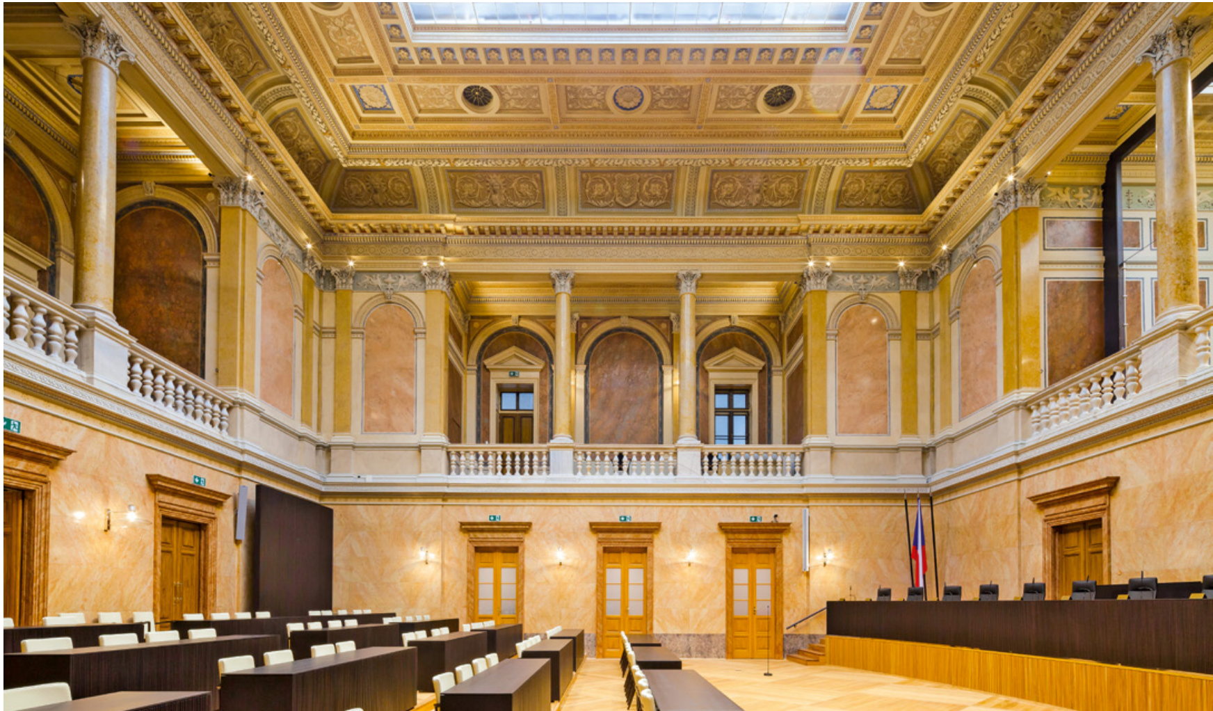
Removal of barriers in the Assembly (Plenary) Hall, which was originally designed in a tiered manner. The staircase was partially removed during the renovation and places for persons with physical disabilities were created in the first row.
