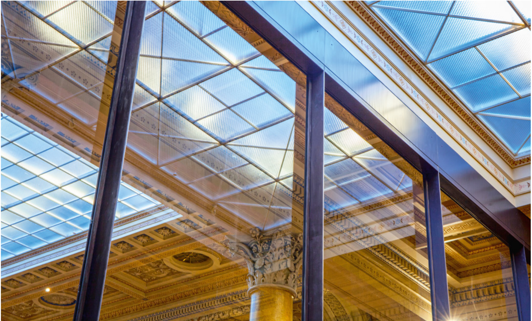
The restored roof light of the Assembly Hall
