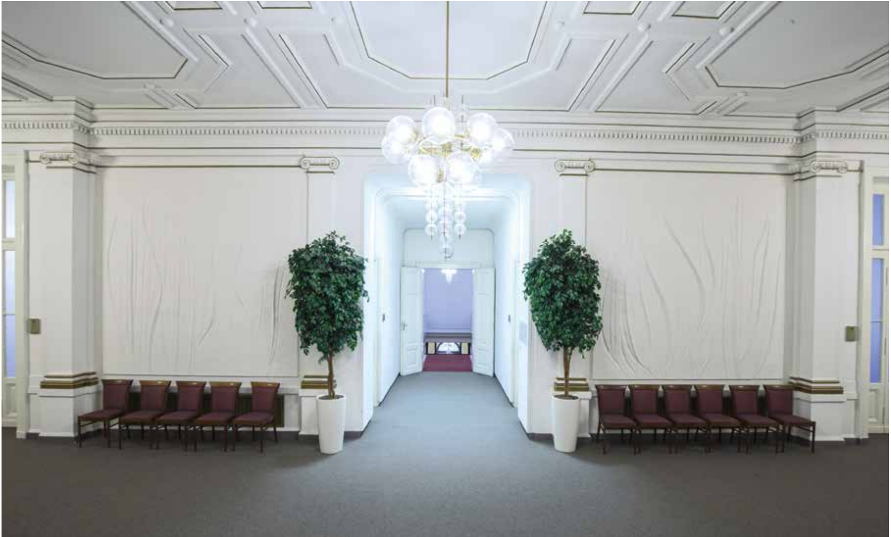
An entrance to the Vestibule of the Assembly Hall before restoration
