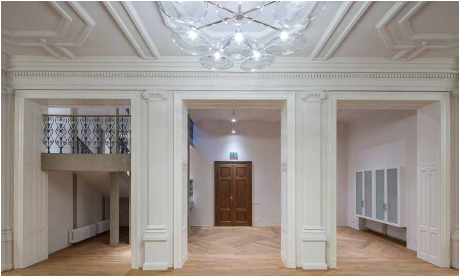
An entrance to the Vestibule of the Assembly Hall after restoration
