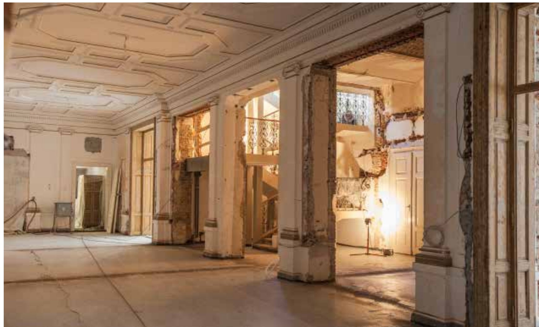
The Vestibul of the Assembly Hall in the course of reconstruction works
