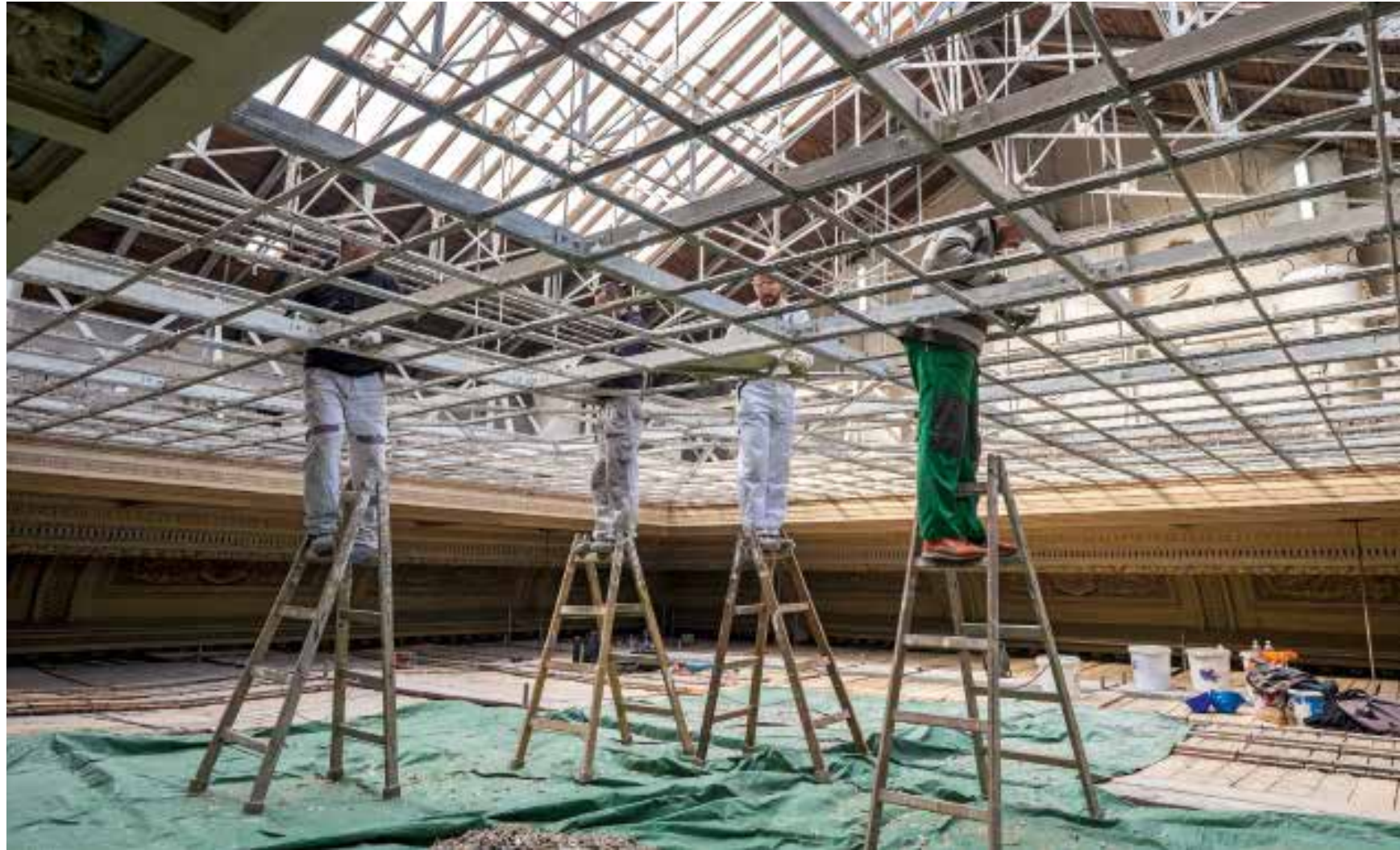
Renovation of the roof light's metal structure
