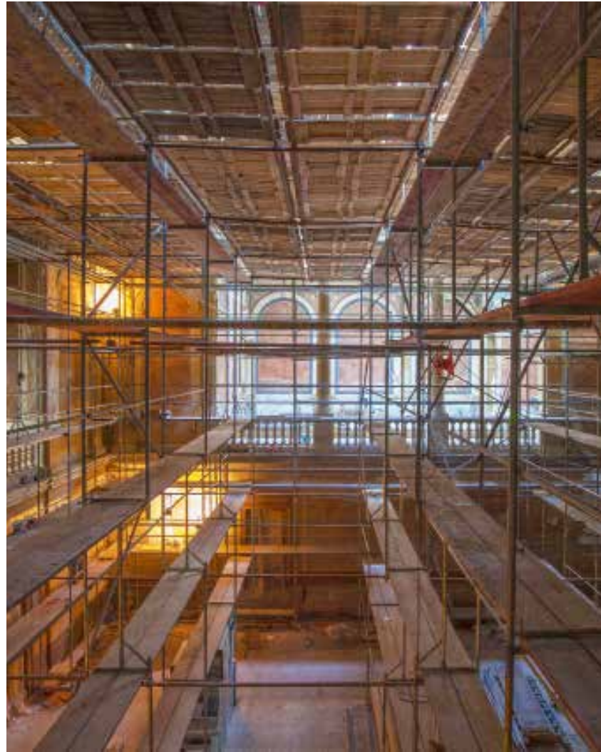
The Assembly Hall in the course of reconstruction works
