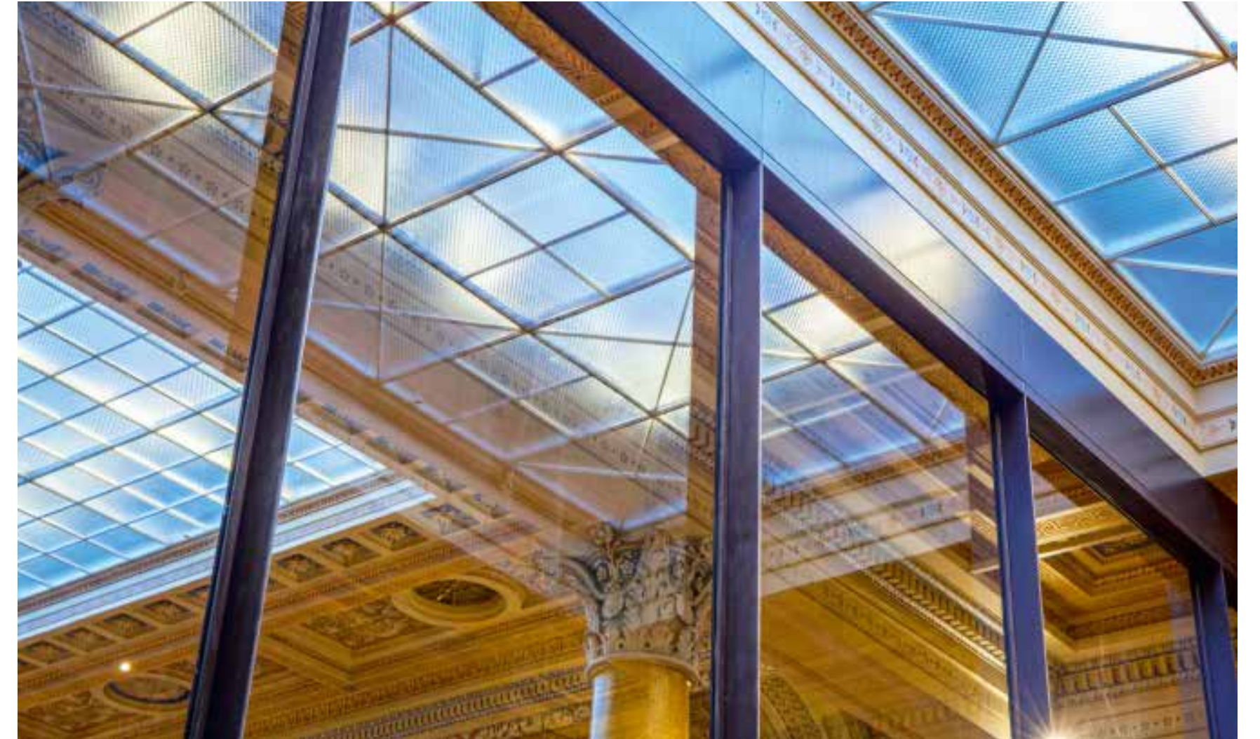
The restored roof light of the Assembly Hall
