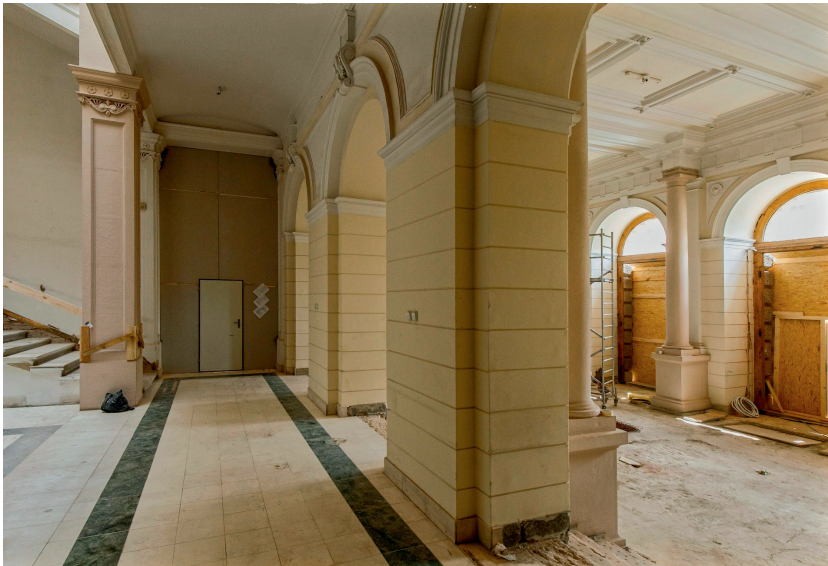
The foyer undergoing the reconstruction
