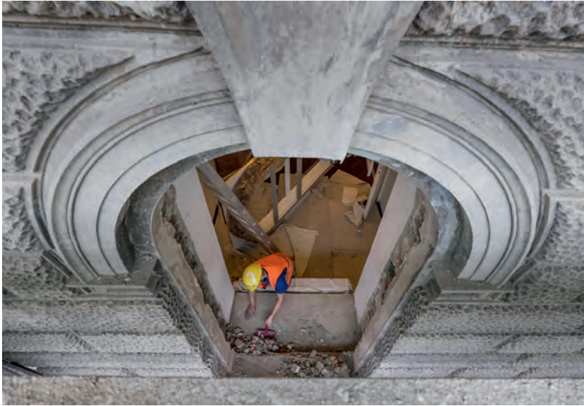
Window block replacement
