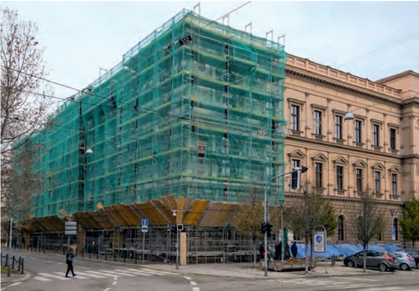
Scaffolding grew quickly on the western facade of the Court © Constitutional Court/Aleš Ležatka
